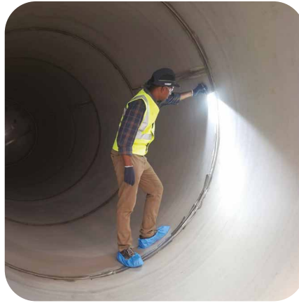
Cleaned for oxygen service for all tanks
